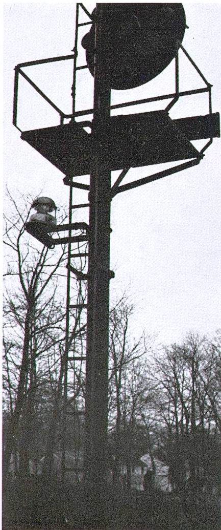
Rotating white beacon below signal head lights to alert crews.
